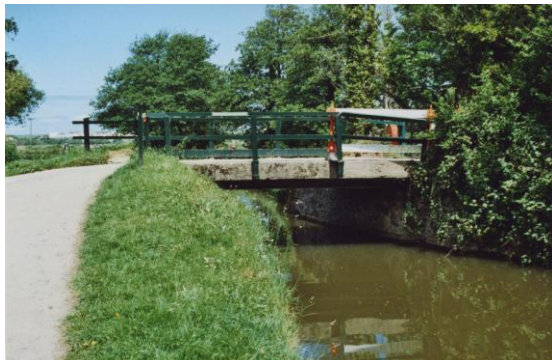
Fig 5. Rodds Bridge - Any new bridge must have sufficient headroom for navigation
