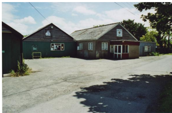
Fig 8. Higher Wharf - Existing buildings
